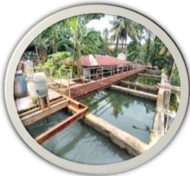
Pengolahan Air/ Water Treatment
